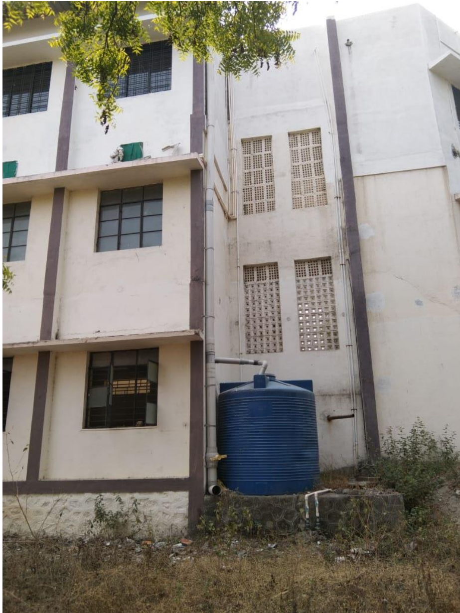
Rain water harvested at Tank
